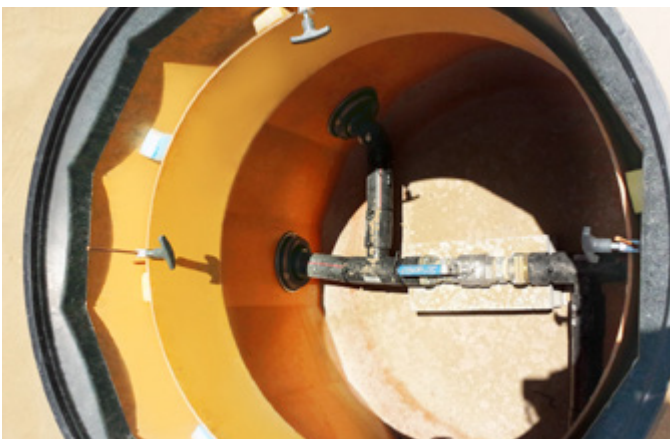
Vacuum testable Fibrelite pipe sealkits form watertight seal
