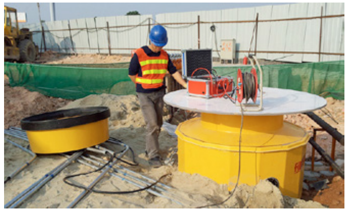
Vacuum tested tank sumps
