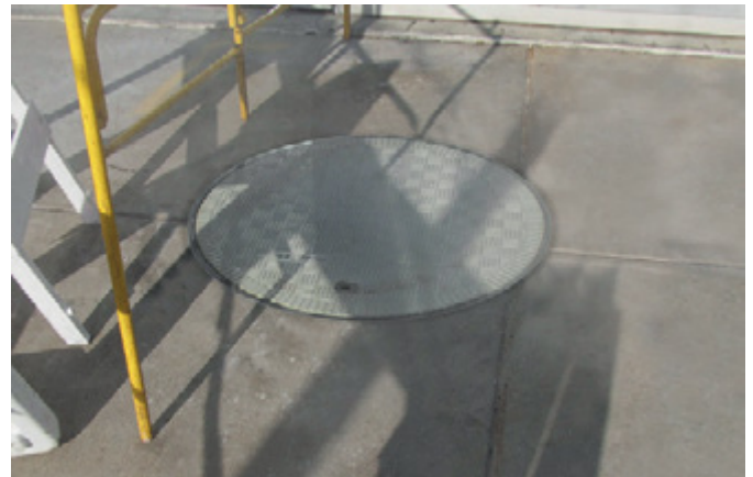
Fibrelite F95 composite cover installed in frame
