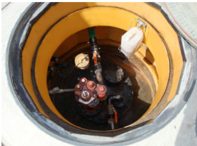
Fiberglass turbine sump with 55" tank collar
