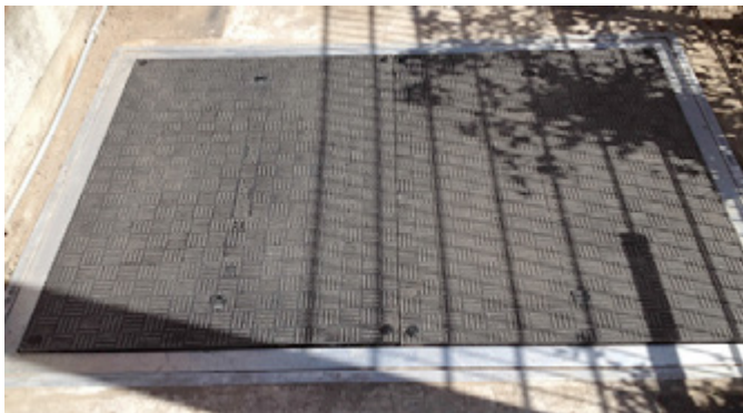
Sealed odour-tight covers installed
