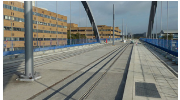
Fibrelite covers needed to be manufactured to work with pre-installed chamber systems
