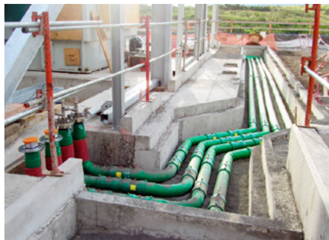
OPW provided a compact solution combining KPS piping and Fibrelite sumps
