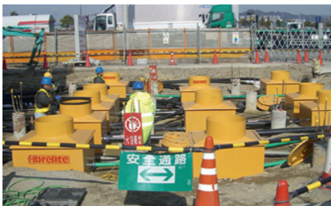
Vacuum tested tank sumps
