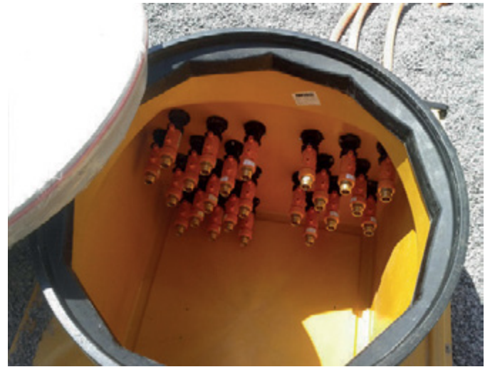
Cable drawpit with 32mm conduit piping
