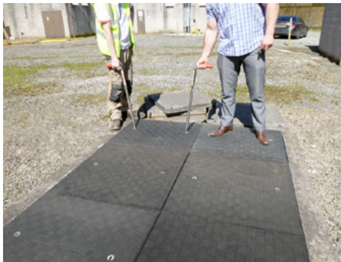
Fibrelite manufactured trench covers which were lightweight and maintenance free
