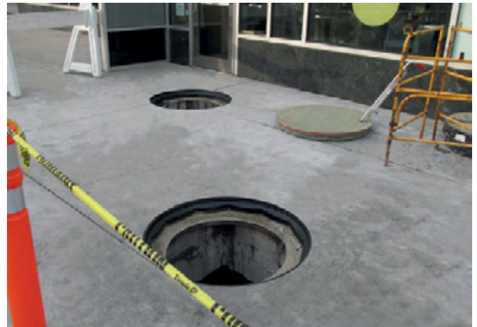
Fibrelite F95 composite cover installed in frame
