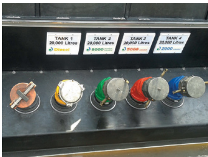
Fibrelite's fuel resistant Viton entry boots
