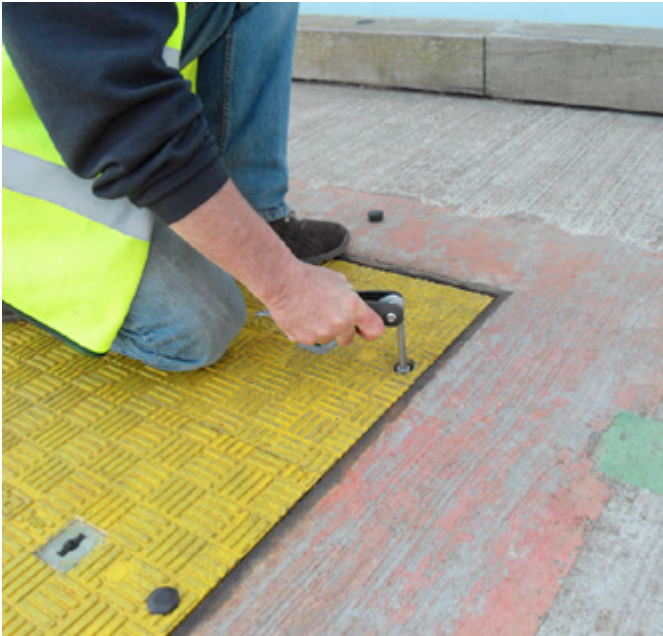
Operator removing the Fibrelite securing system
