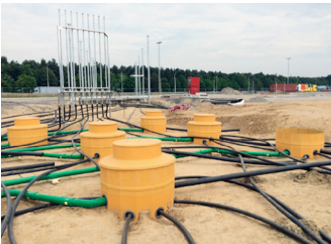
Fibrelite chamber systems are fully vacuum testable and watertight
