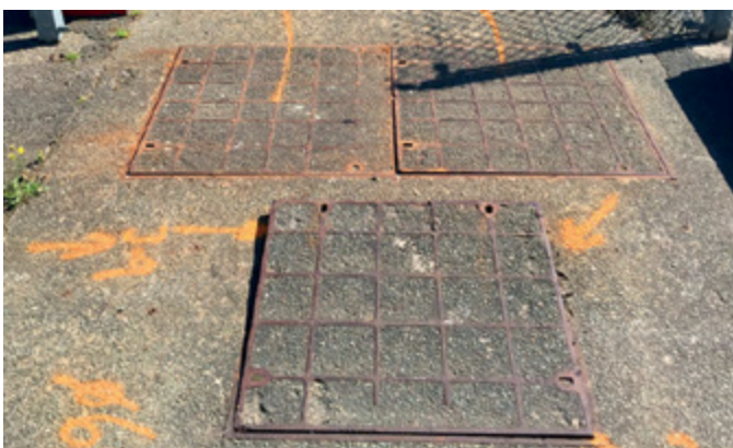
Previously installed heavy concrete recess covers
