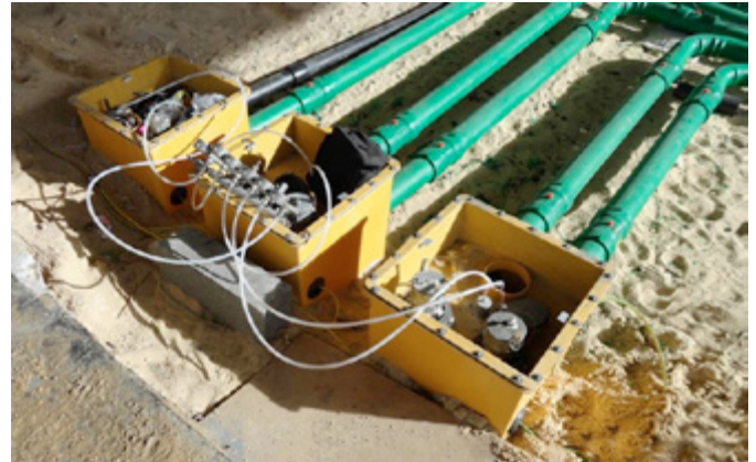
Secondaryly contained Fibrelite remote fill sumps
