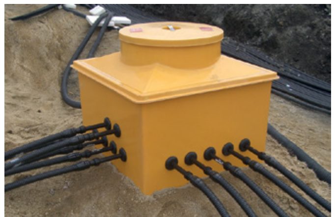
Fibrelite's electrical conduit drawpit being installed
