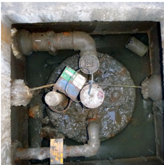
At this site, the old tank upstands were too small for the traditional bolt down tank sumps / chambers
