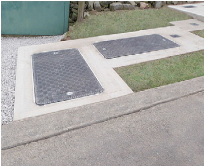
The 25 tonne load tested lightweight covers
