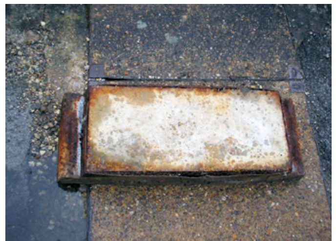
Corroded previously installed cover hinge
