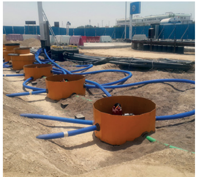
Fibrelite tank sump system with pipework attached using Fibrelite pipe entry sealkits, forming a watertight seal
