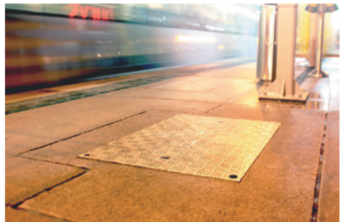
Fibrelite's lightweight securable composite covers
