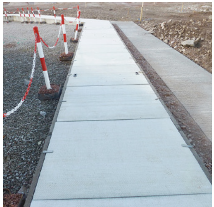
Concrete covers unable to withstand pedestrian traffic
