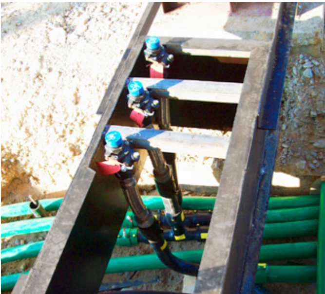
Sinooil required a solution that allowed emergency valves to be installed under dispensers
