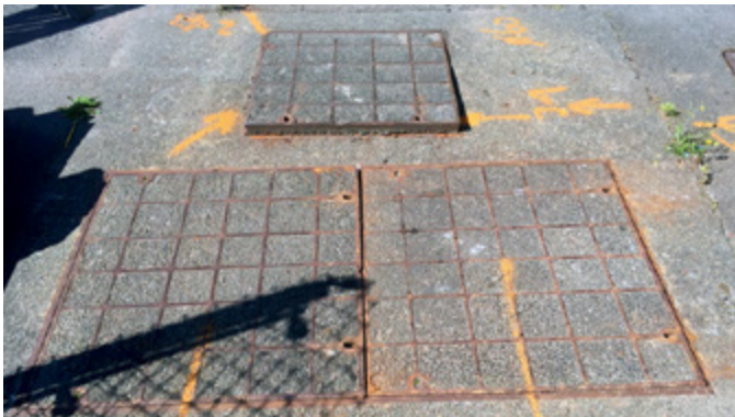
Covers were showing signs of severe corrosion
