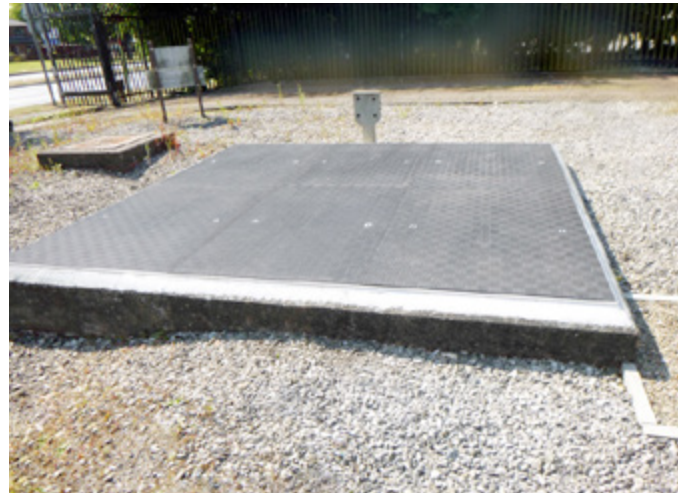
Covers can be easily, quickly and safely removed using Fibrelite's FL7 lifting handles
