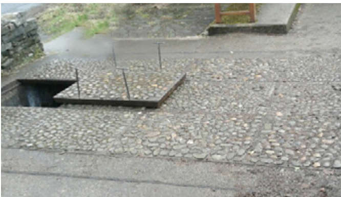
Cobbled covers requiring lifting equipment
