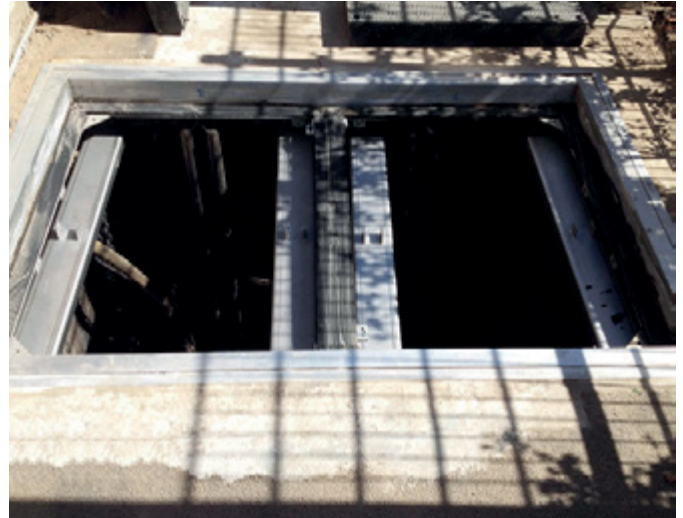
Removable centre beam supports covers
