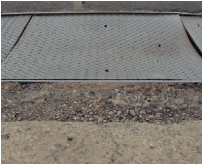
Corroded and deformed cheap steel covers
