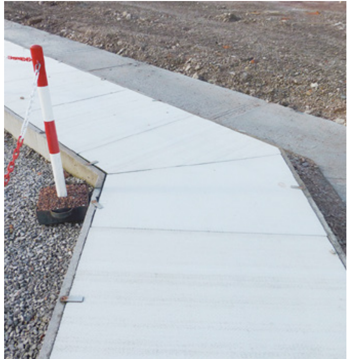
Previously installed low quality concrete covers
