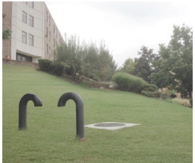
Fibrelite lightweight composite cover
