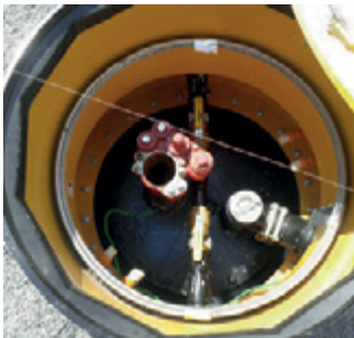
Fibrelite's 1.2m 16 sided turbine sumps being installed
