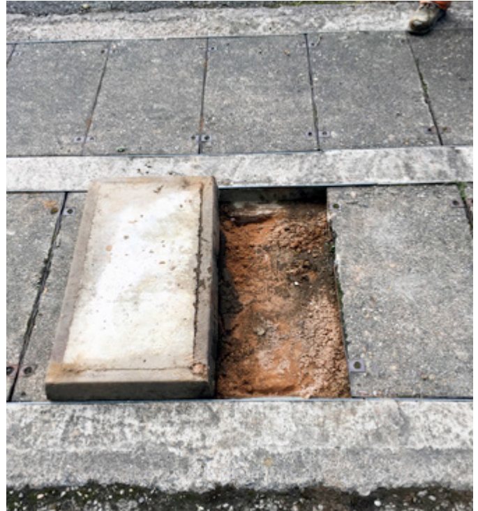
The previously installed covering arrangement was deteriorating
