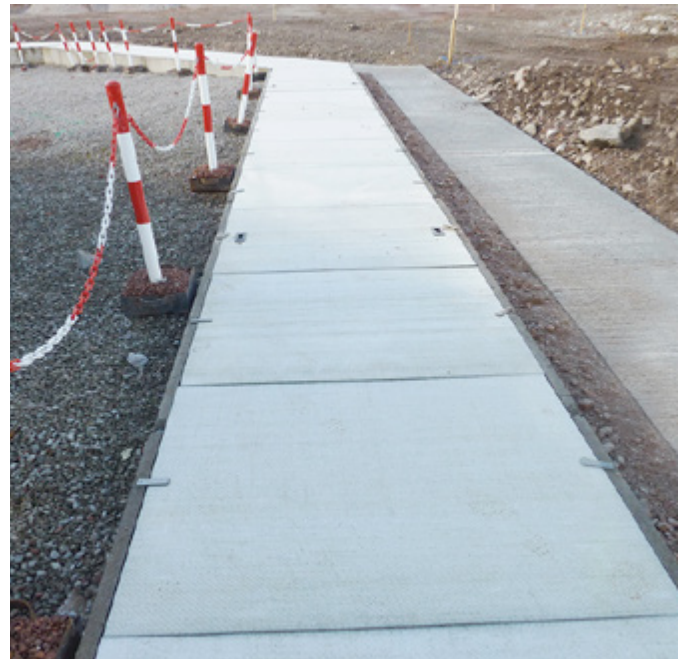
Concrete covers unable to withstand pedestrian traffic
