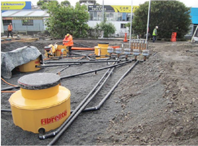
Fibrelite sumps are vacuum testable ensure watertightness
