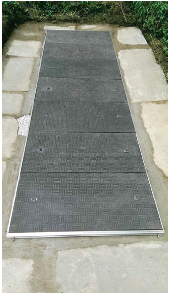
Chemically inert and corrosion resistant covers
