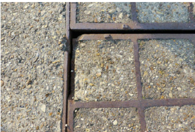
Corroding previously installed covers
