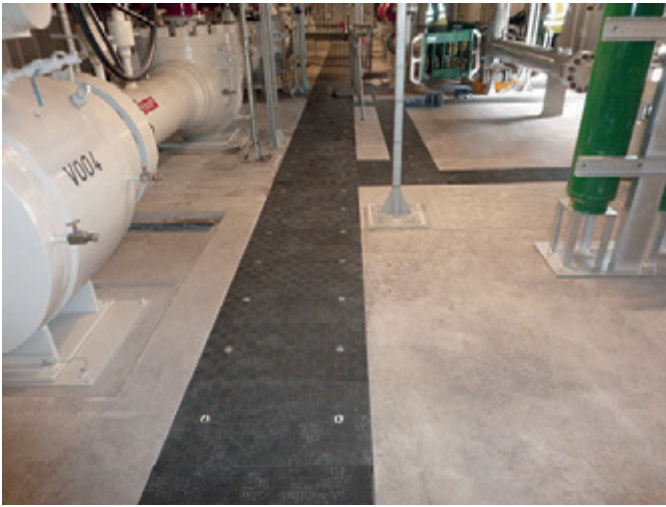
Non slip coating is applied to the top of the panels
