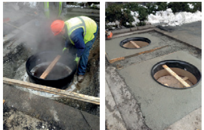
Fibrelite installations are simple – a fibreglass skirt can be used as a preform and to set the frame at grade
