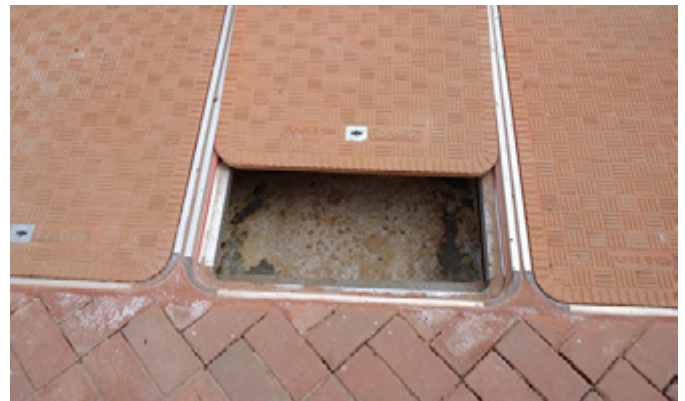
Fibrelite's odour tight composite covers
