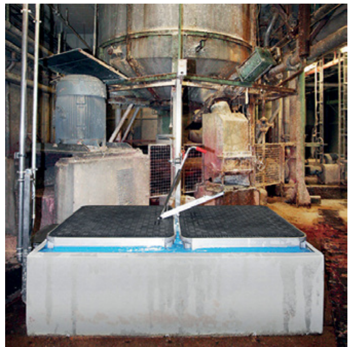
Complete installed Fibrelite covers
