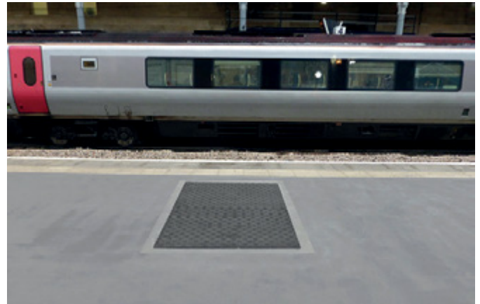
Lightweight Fibrelite covers now installed on platform
