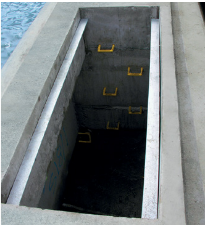
Access pit along edge of quay
