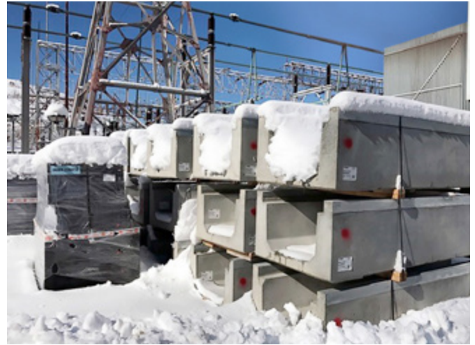
Trenwa's precast trenches ready for installation
