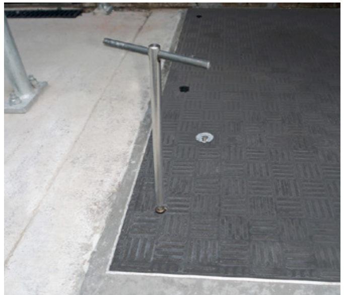
Secured/restrained covers, preventing unauthorised access
