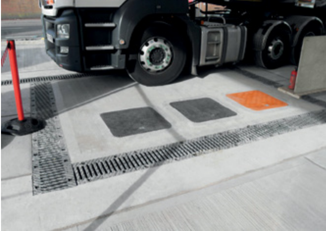
The unique offset sump/corbel arrangement allows for bi-lateral pipe exits
