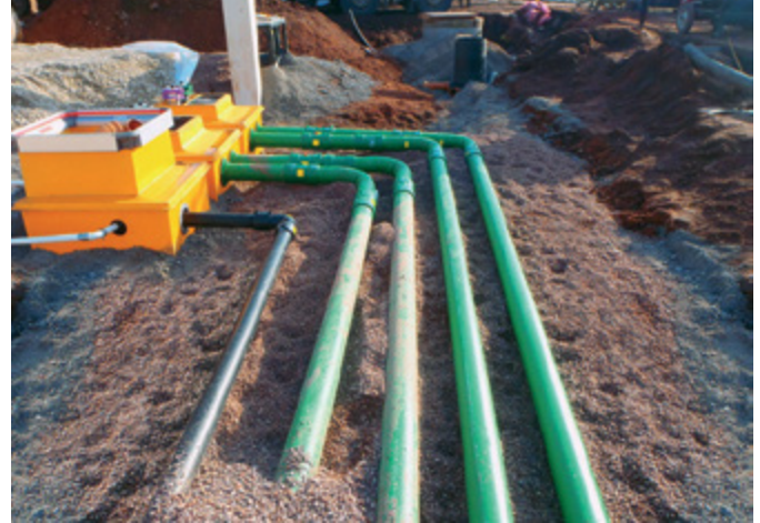
All integrated KPS fittings weld both pipe walls simultaneously
