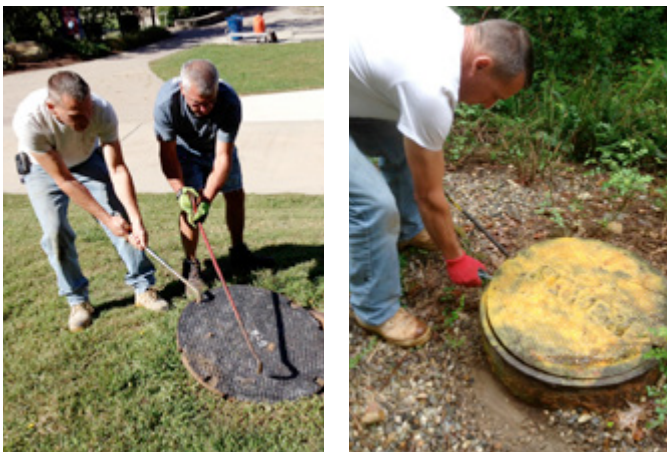
Heavy cast iron covers pose a significant threat of back & shoulder injuries along with the risk of trapped extremities
