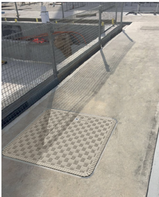
Installed cover over balance tanks
