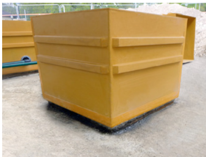
Fibrelite tank sump mounted on old tank upstand
