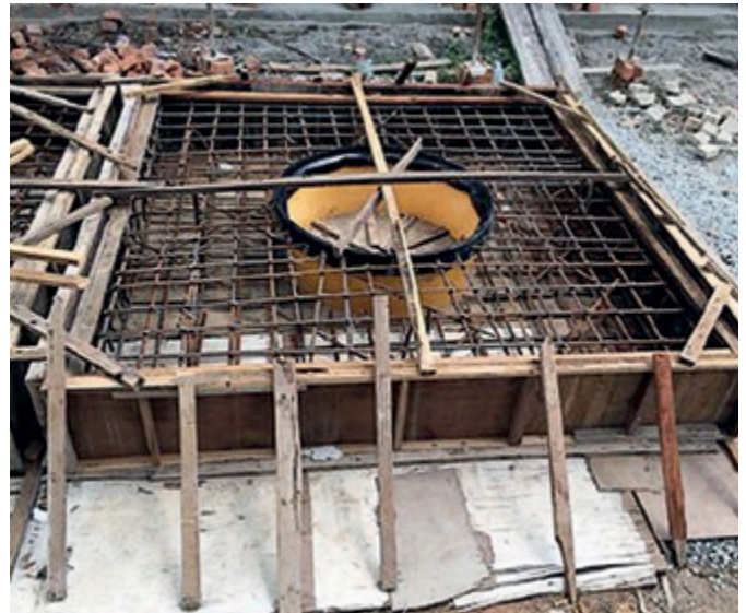
Prefabricating concrete plinth with Fibrelite FL90 frame
