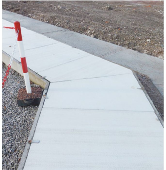
Previously installed low quality concrete covers
