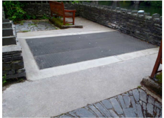
Lightweight Fibrelite trench covers now installed
