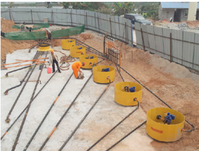
Fibrelite tank sumps (S14-390) being installed
