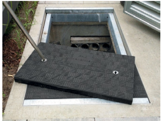
Fibrelite trench panels installed over the chamber
