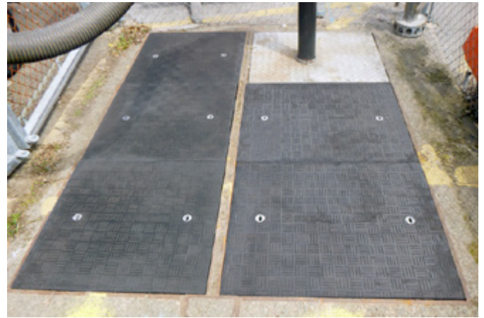
Fibrelite covers allow safe removal by hand
