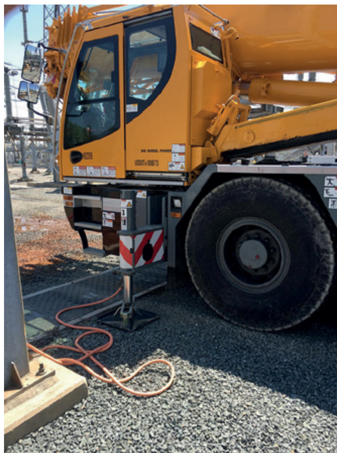
HS-20 load rated trench covers are strong enough to handle an 18 tonne load
