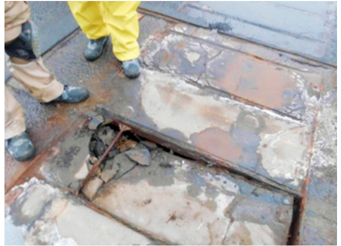
Heavily corroded previously installed covers
