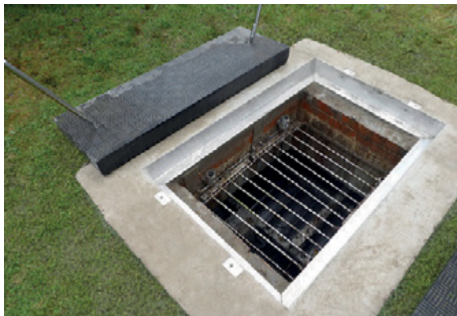
Safe and easy manual removal: Fibrelite FM45 covers are removed by hand from the CSOS (Combined Sewage Overflow System) chamber
