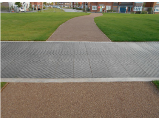
Fibrelite's treads incorporate a specialised anti-slip material for added safety
