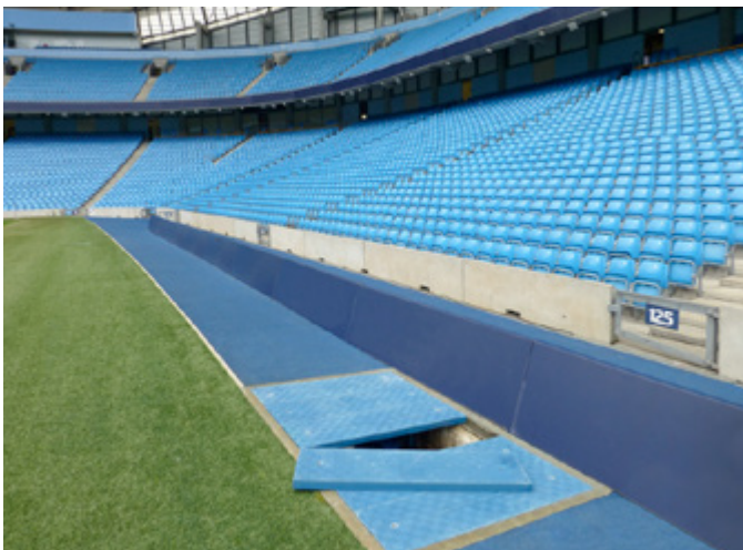
Fibrelite trench covers have an anti-slip surface
