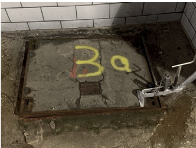
Old unsafe concrete covers
