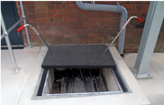
Sealed Fibrelite covers prevent water ingress
