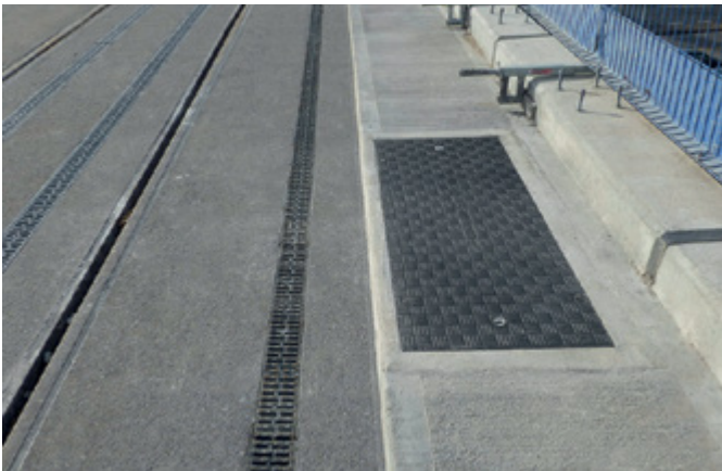
Bespoke trench covers for trackside gear
