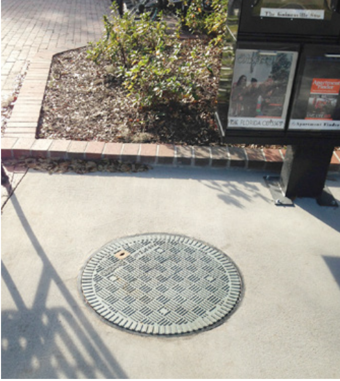
Lightweight composite steam cover - product code F65
