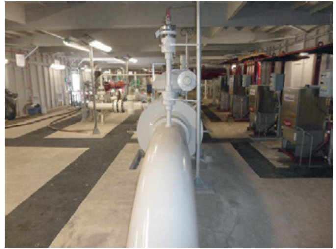
Longer length trenches with no additional support
