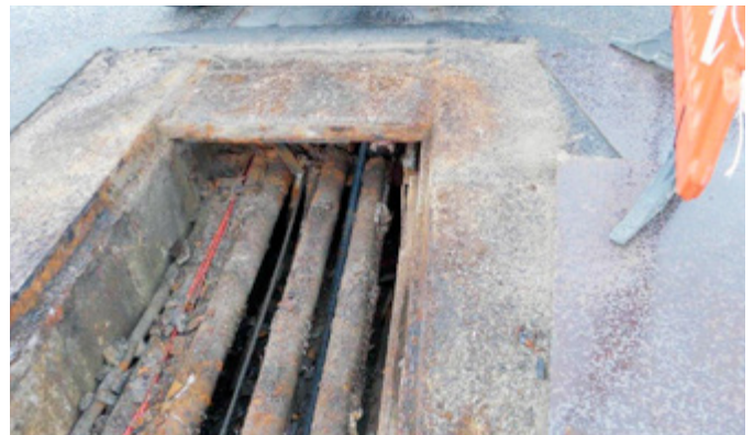
Previously installed failing concrete and metal covers
