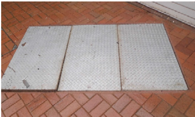
Previously installed odour-emitting galvanised covers
