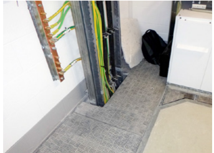
Fibrelite covers are maintenance-free and corrosion resistant
