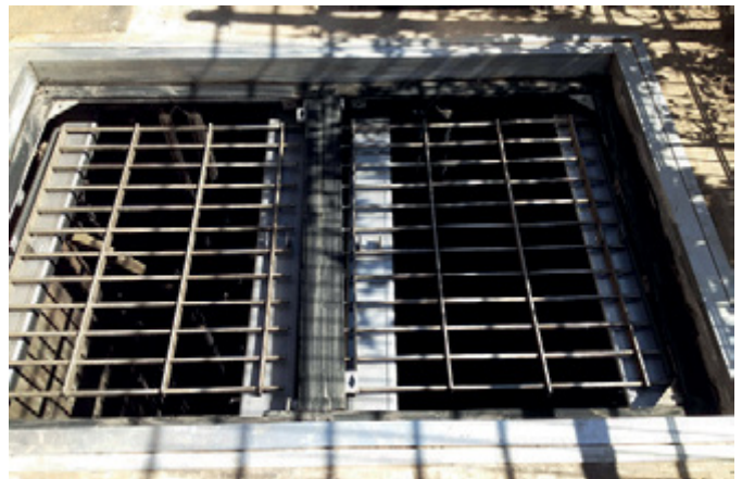
Removable beams hold safety grid
