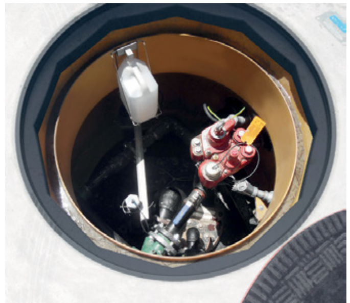
Fibreglass 1.2m (42") turbine sump
