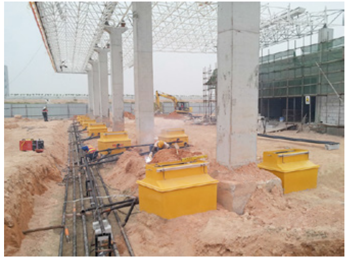
Fibrelite's Gilbarc/China EL-GC-T05403-SH10 dispenser sumps
