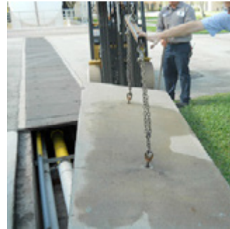
Traditional concrete panels are unsafe and labor intensive to remove and often break apart over time
