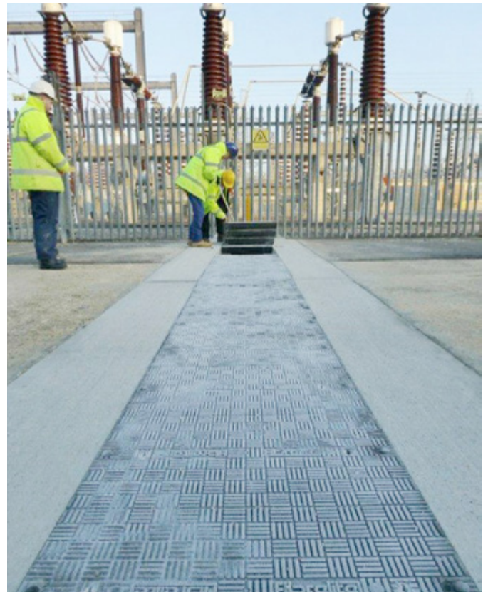
Fibrelite covers provide safe easy access to electrical cabling
