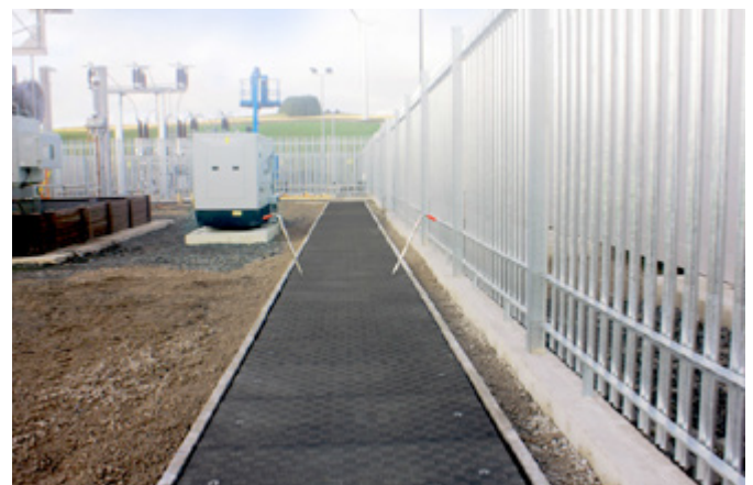
Bespoke Fibrelite trench covers 1250mm span
