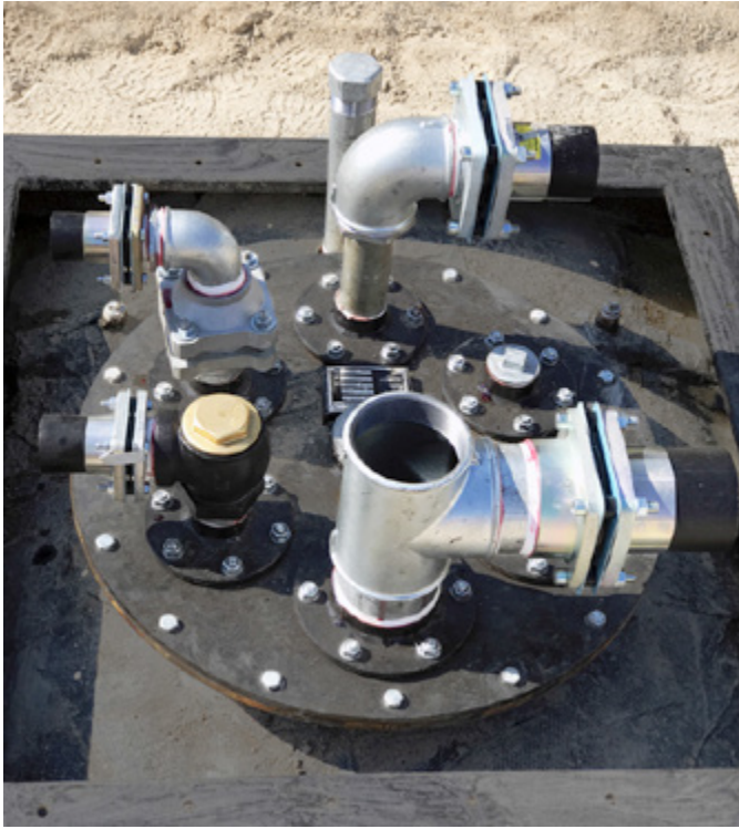
OPW 14NL angled check valve allows manual fuel flow control
