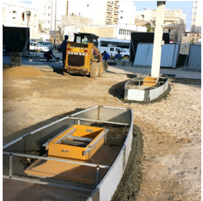
Fibrelite EL-G-E500 dispenser sumps ready for concreting
