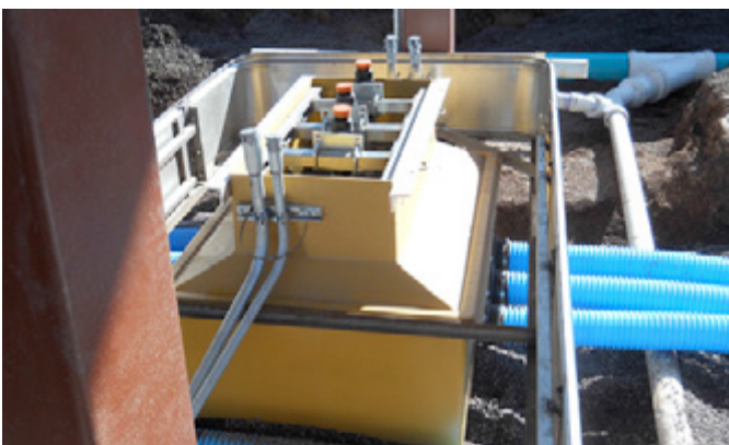
Fibrelite's E85 compatible Encore 500 dispenser sumps
