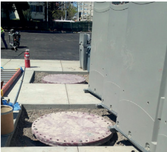
Fire manway lids (tank buried underneath)
