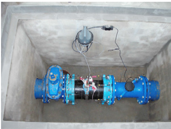
Underground water monitoring system (Image credit: Aguas de Cádiz)
