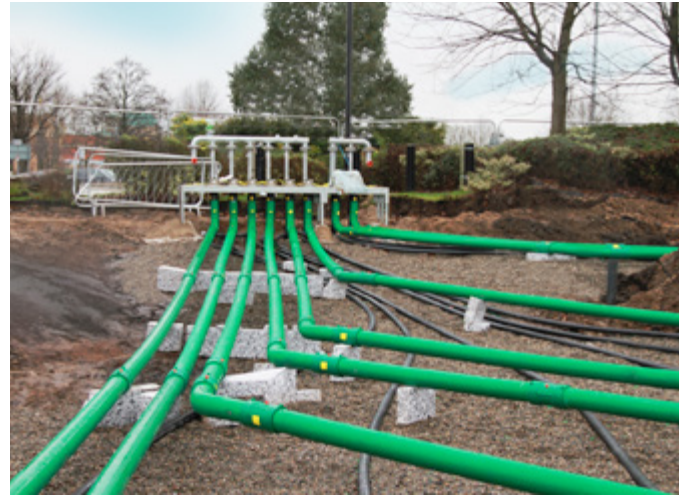
KPS formed bends below fill point
