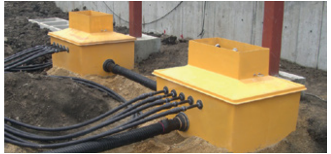
Fibrelite's Tokico AB26L dispenser sumps
