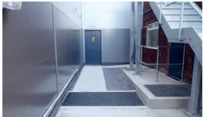
Retrofitted sealed Fibrelite covers installed
