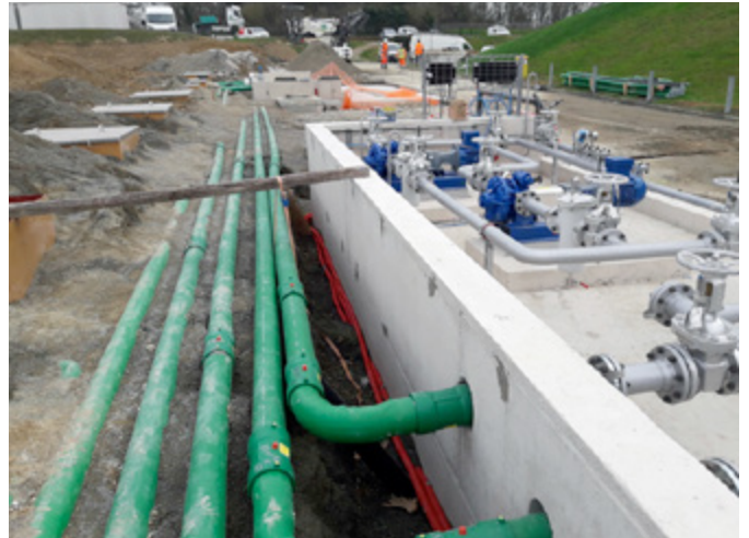
KPS conductive double wall piping provides the highest possible level of safety for Ethanol's potential to generate chargee
