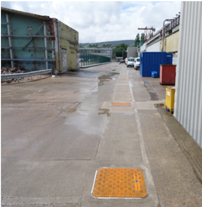
Heavy duty Fibrelite FL60/D400's
