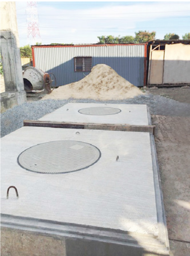
Plinths ready for installation
