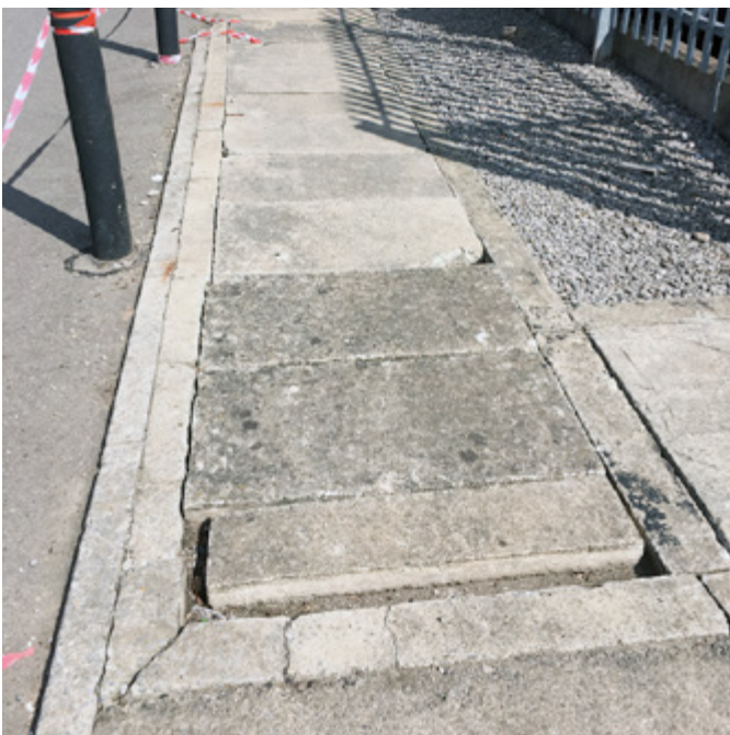
Previously installed failing concrete trench access covers
