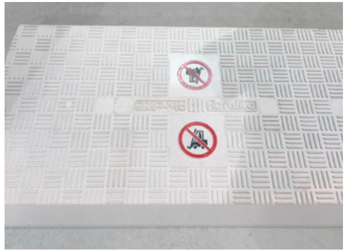
Custom FRP composite trench covers manufactured to fit into existing rebate
