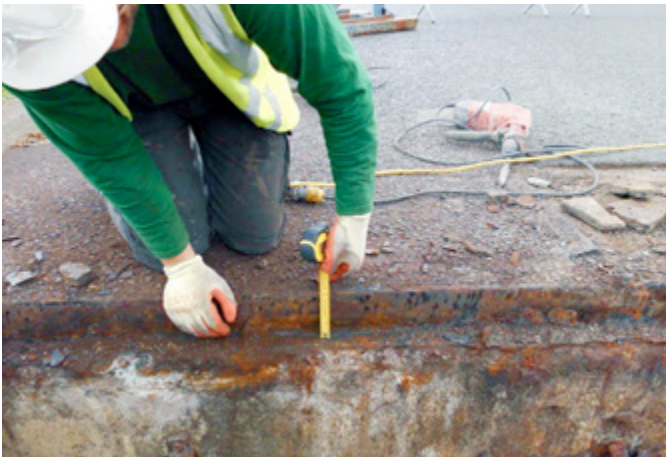
Previously installed heavily corroded access covers
