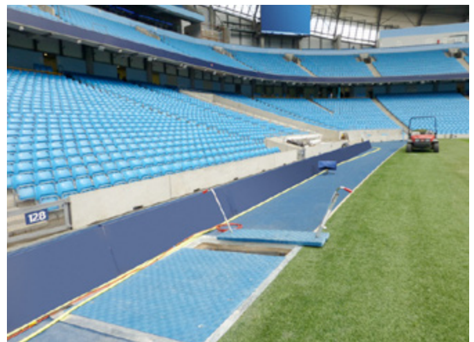
The Fibrelite trench covers and ergonomically designed lifting aid allows for a safe and easy removal
