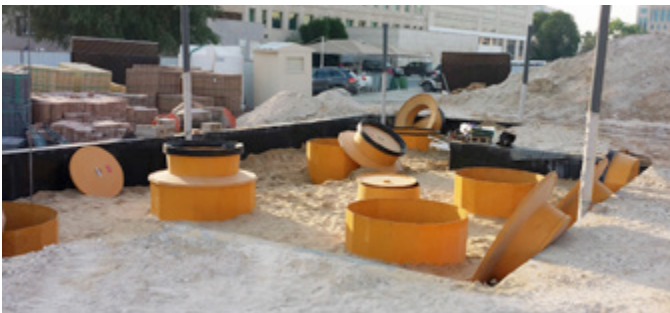
Fibrelite S14-390 tank sumps under installation
