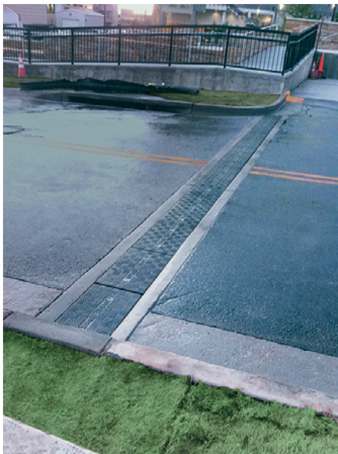
Fibrelite covers offer a clean lightweight alternative to heavy and iron concrete covers
