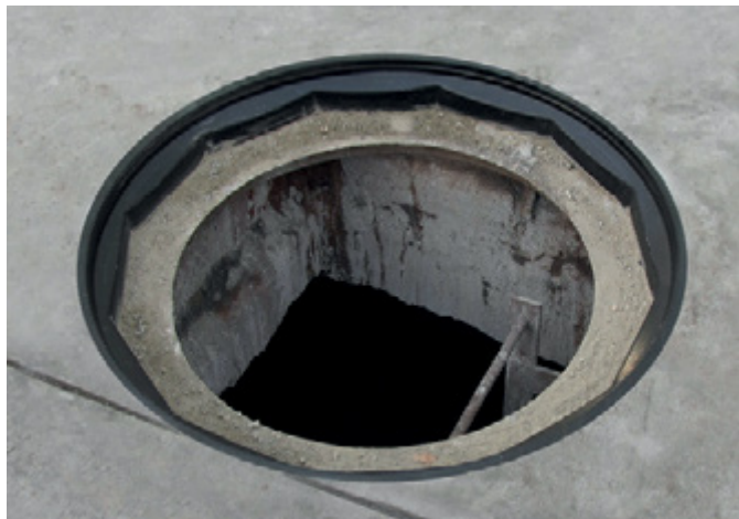
Fibrelite composite frame installed in sidewalk
