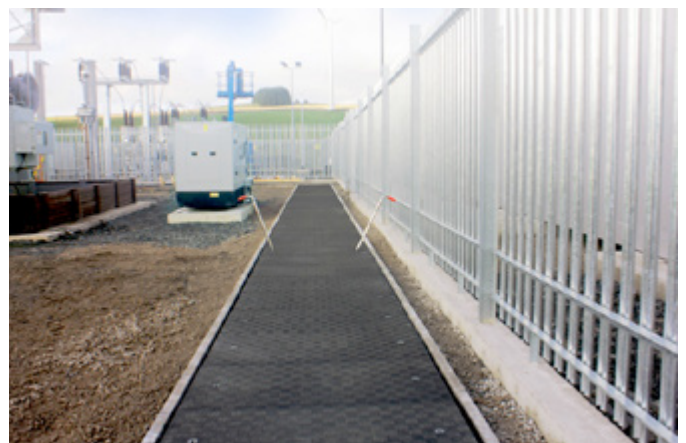
Bespoke Fibrelite trench covers 1250mm span
