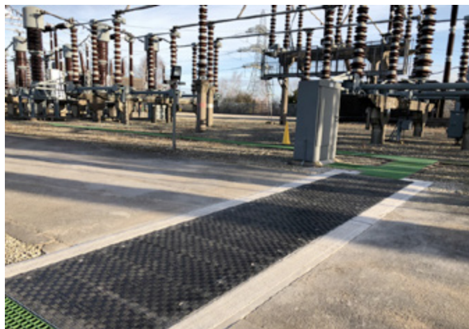
Fibrelite covers and frames were designed to fit existing apertures
