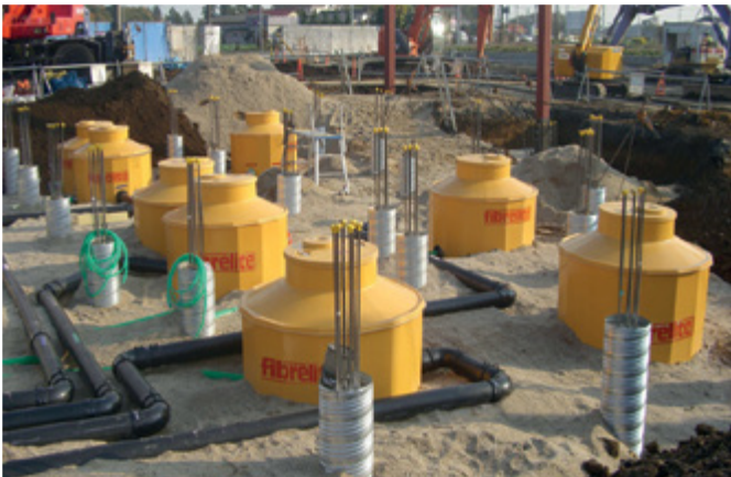
Fibrelite's 1.4m 16 sided tank sumps being installed
