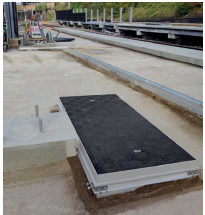
Fibrelite FM45-B125 trench cover
