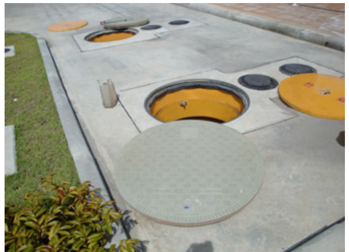
40" (1020mm) Fibrelite cover (FL 100) with 25 tonne load rating
